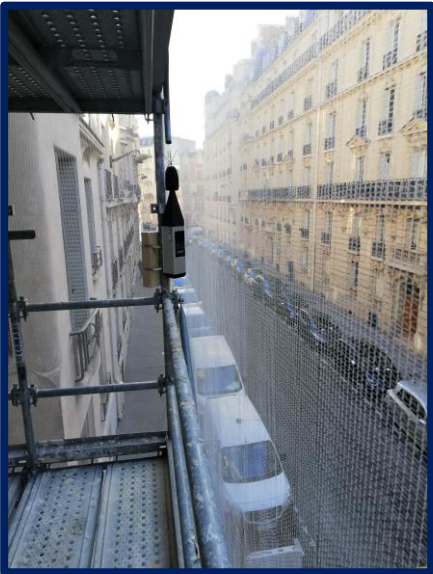
CONSTRUCTION SITE FENCE / PROPERTY LIMIT
